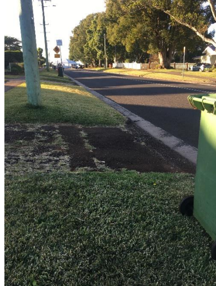
Photo taken on Wardell Road towards the Driveway Servicing 17 Wardell Road
